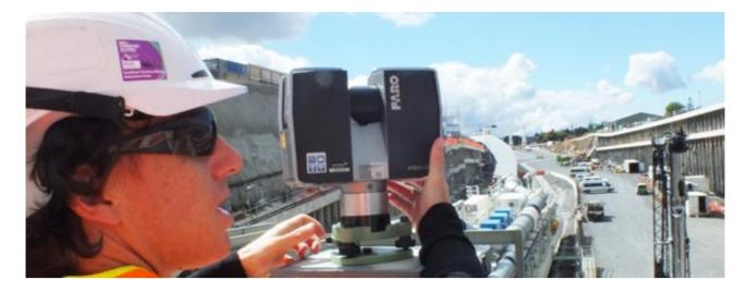
Surveyor Mike Cutfield of Fletcher Construction has been utilising a FARO Focus3D high speed laser scanner for monitoring work around the tunnel portals on the enormous Waterview Connection 'Roads of National Significance' project in Auckland. Click on more information to see how they faired...
